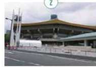
The Nippon Budokan was completed in 1964 with the aim of popularizing the martial arts. At present it is often utilized for entertainment events such as concerts.
